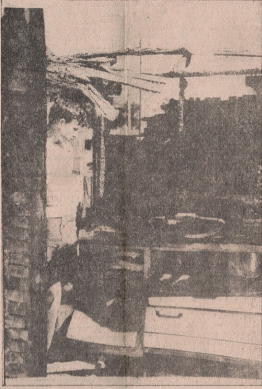
FIRE'S ORIGIN: The charred remains of the Wilcox kitchen at 517 2nd avenue still house the kerosene range which is believed to have started the fire early this morning. Kenneth Wilcox is at left. A five-gallon can of kerosene which was beside the stove is thought to have exploded.
